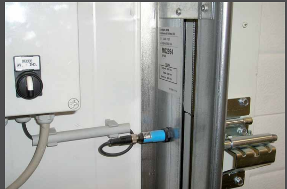
SENSORE PER INTERCONNESSIONE RAMPA-PORTONE DOCKLEVELER-DOOR CONNECTING SENSOR
